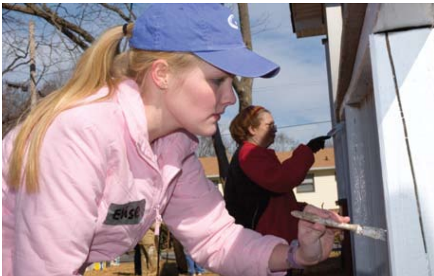
◀ Community service is a high priority for Georgia Tech students such as Elise Mendenhall, an undergraduate Civil and Environmental Engineering major. Mendenhall is pictured painting a house as part of a local Habitat for Humanity project.
