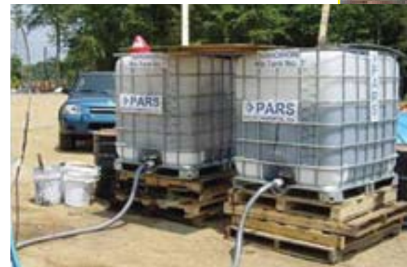
An injection setup for nanoiron slurry.
